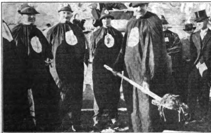
Turning the first spadeful of earth on the site. R. A. Hiscox, Supreme Bojum of Hoo-Hoo and chairman of the building committee of the Board of Governors, handling the wooden spade, made with a fir blade and a sugar pine handle. The earth is to be preserved in a box made of redwood, the "wood everlasting," as it will be handed down to future generations, in the archives of Hoo-Hoo.
